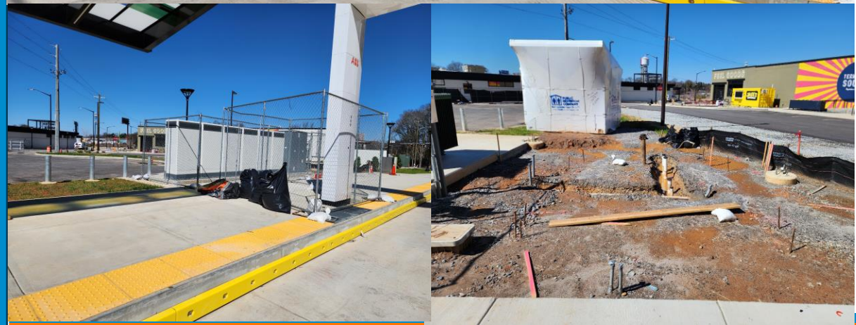
Carver Station – Construction Activities
