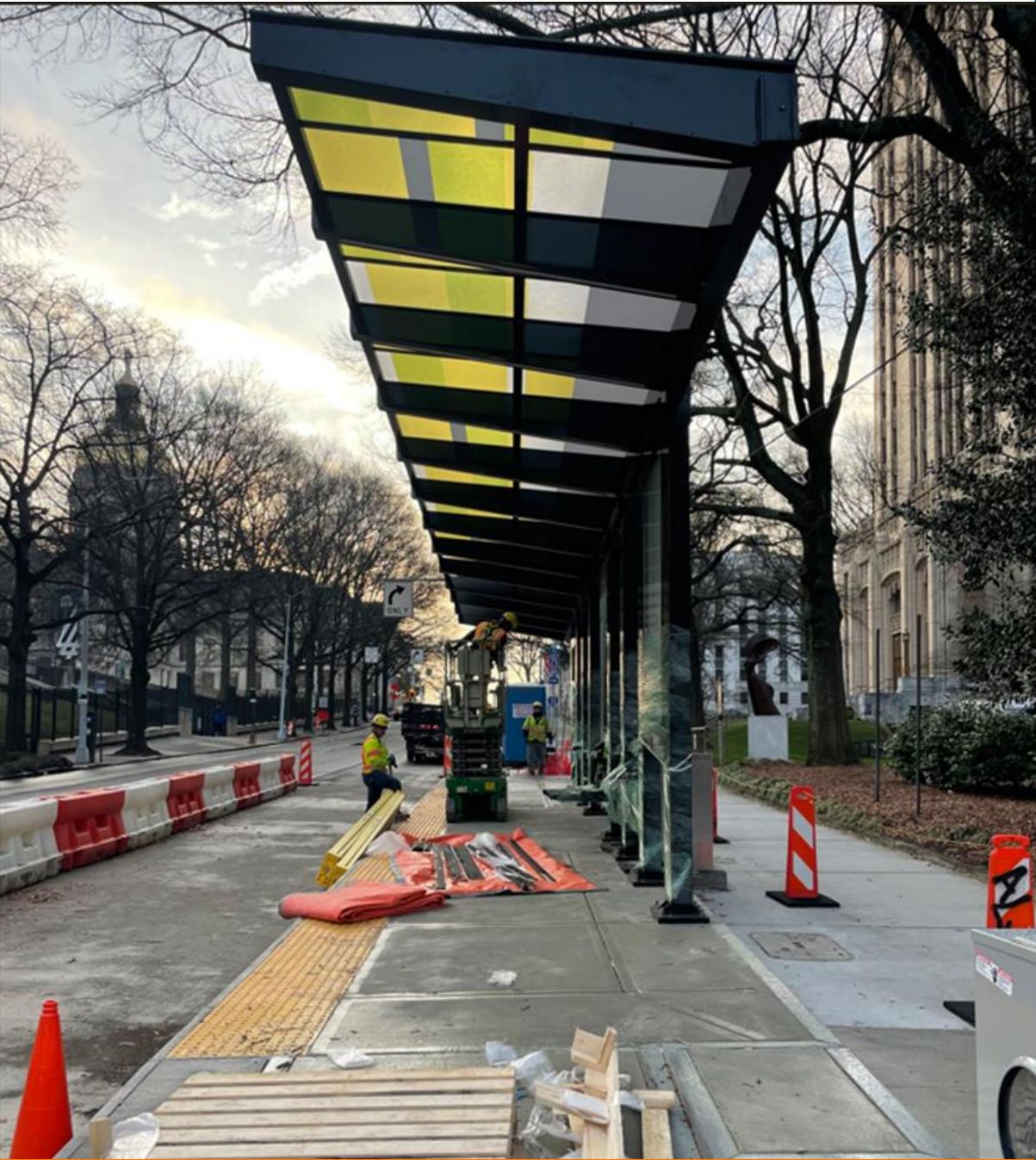
City Hall Station - Shelter Construction
